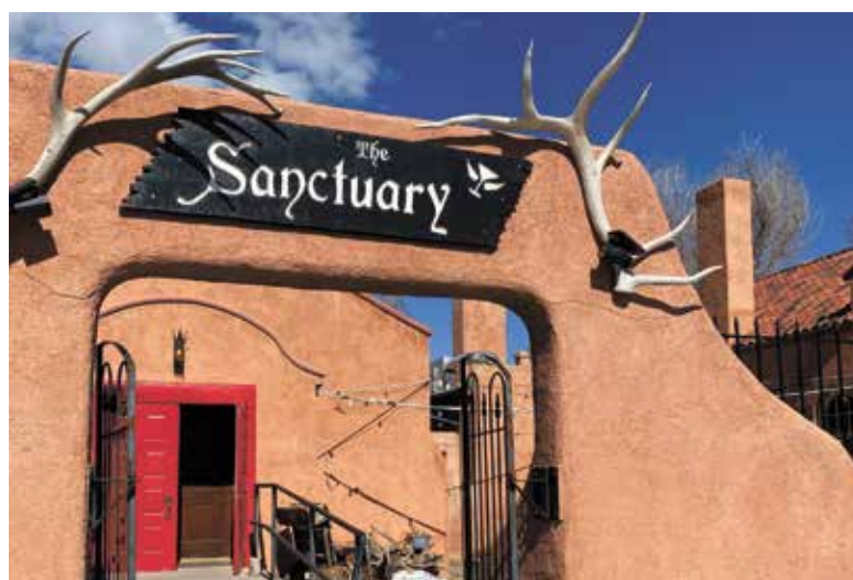
The Sanctuary was created in the footprint of the former historic St. Thomas Episcopal Church in Alamosa.
