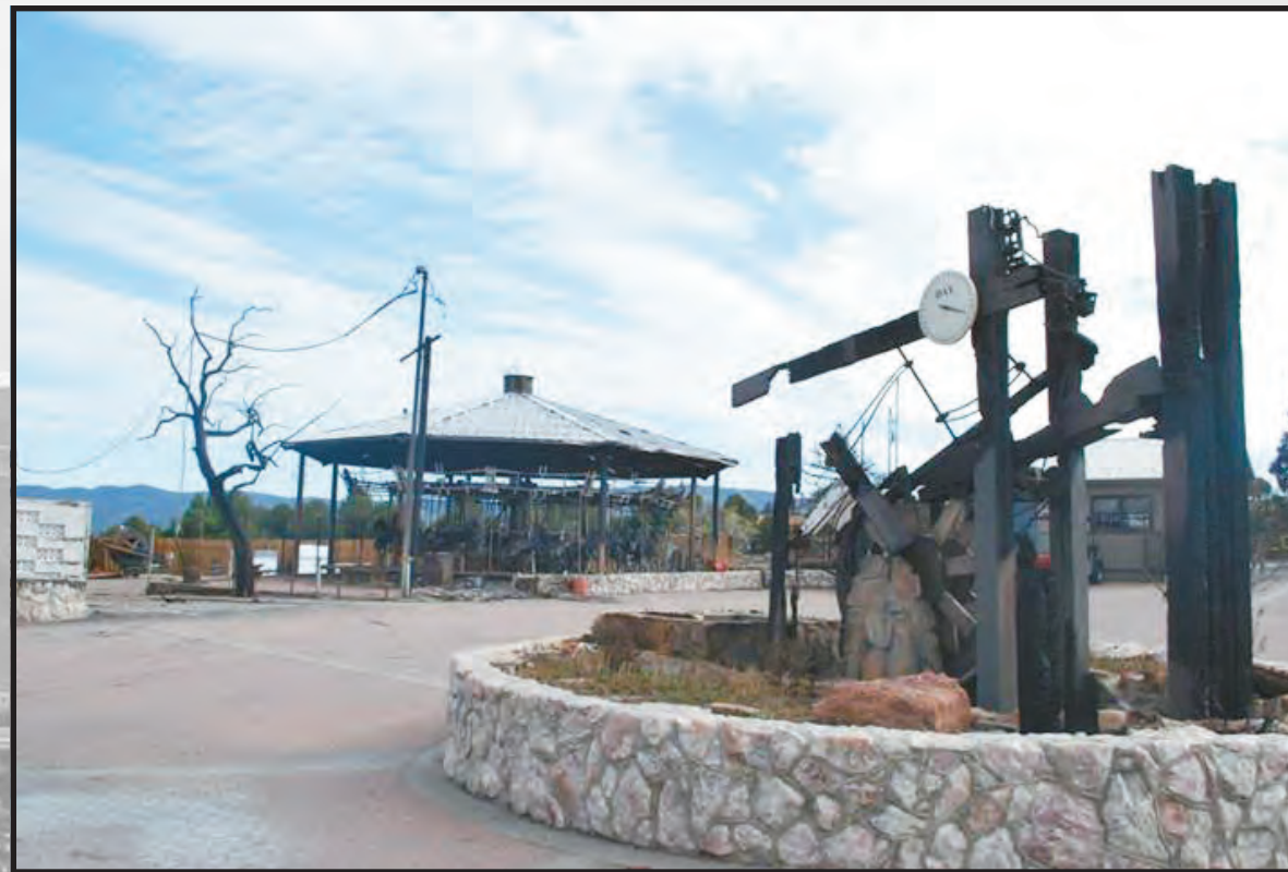
Damage to the antique carousel and water clock.
