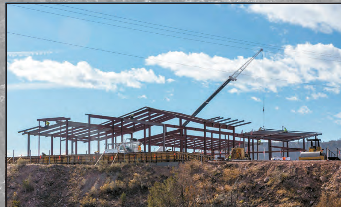
The new Visitor Center under construction.
