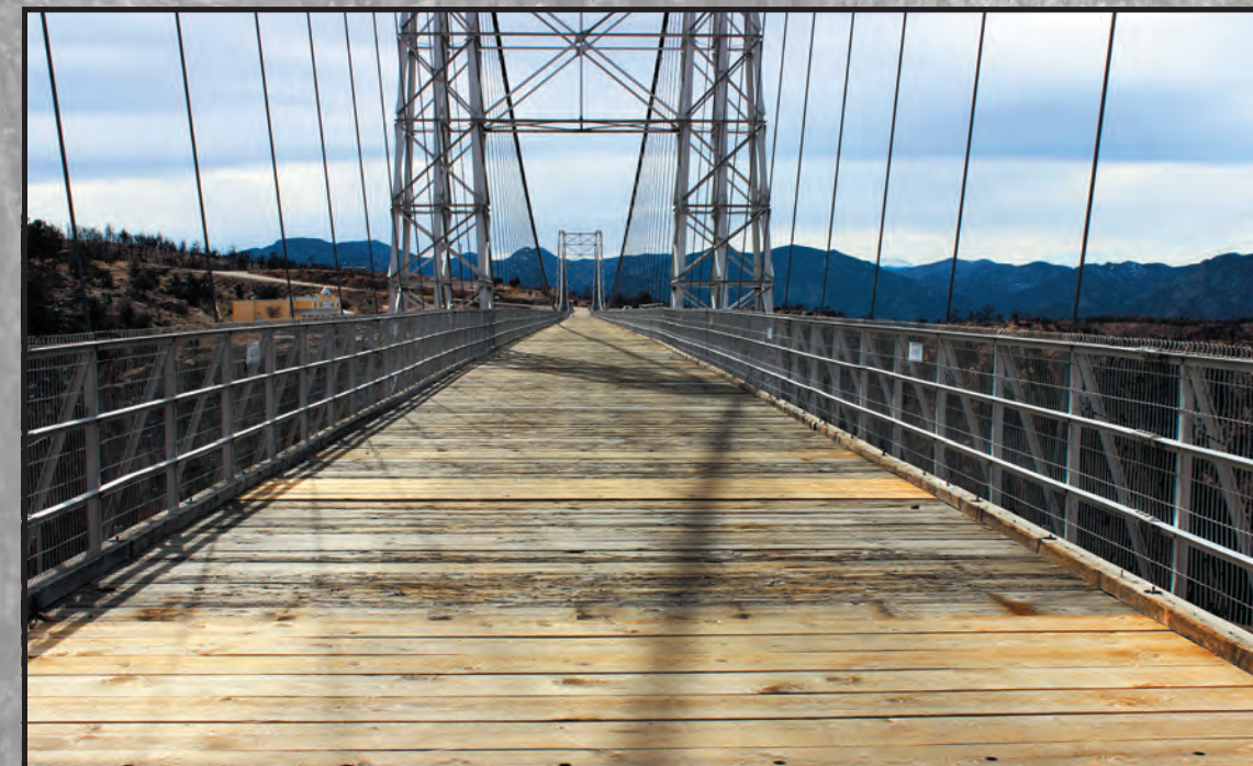
The spectacular bridge sporting new planks.
