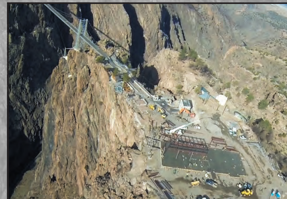
Aerial view of the reconstruction progress.
