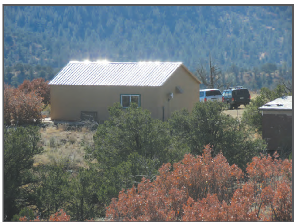
This pot processing building is the building allegedly constructed without a building permit from Fremont County. It is about 60 feet from the Chambers property line.
