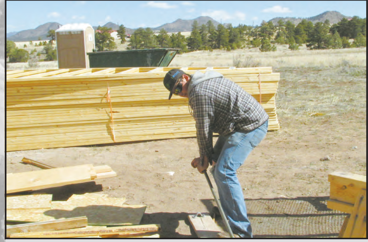
Lind bending rebar.
