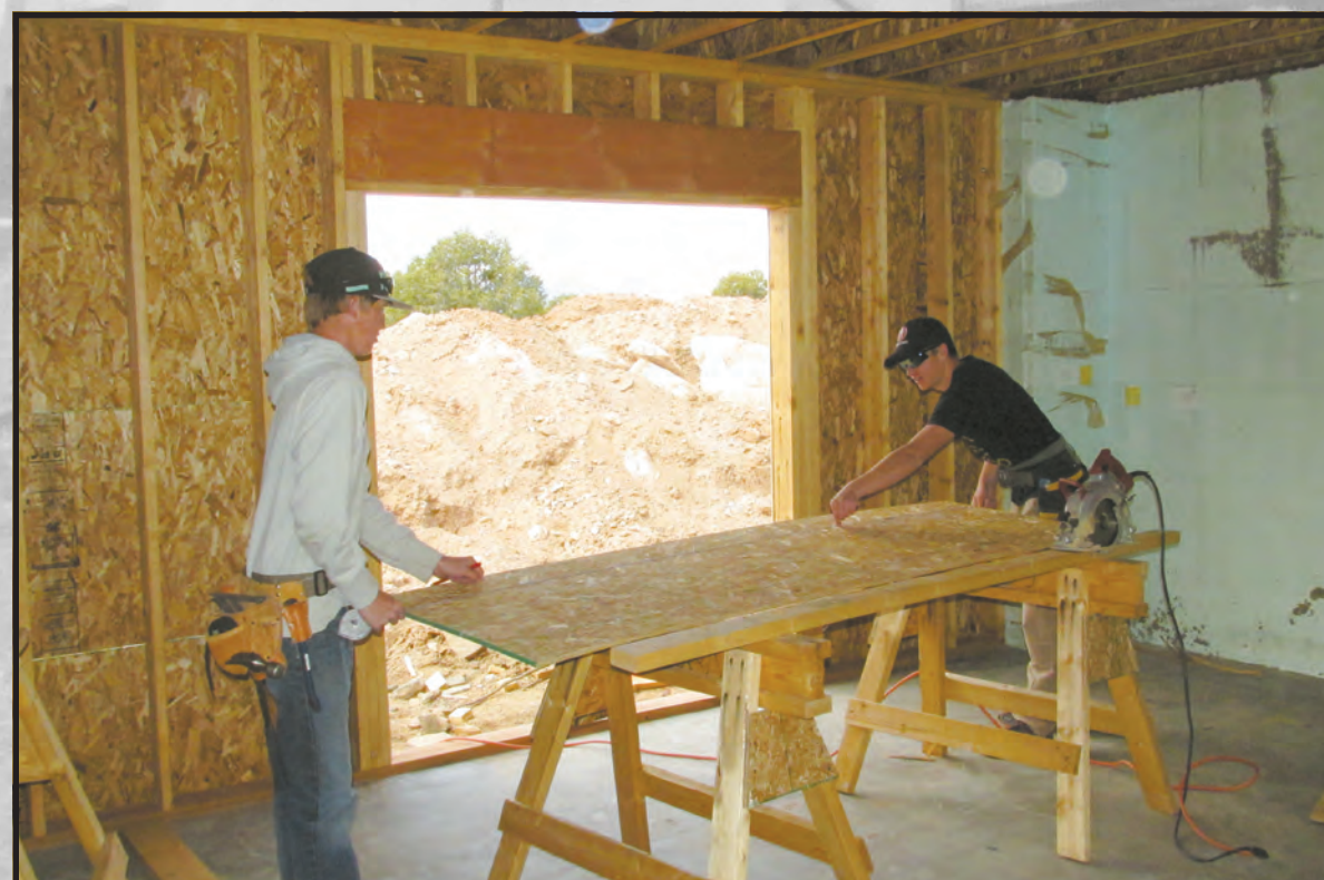
Rusher (left) and Koble measuring for a cut.
