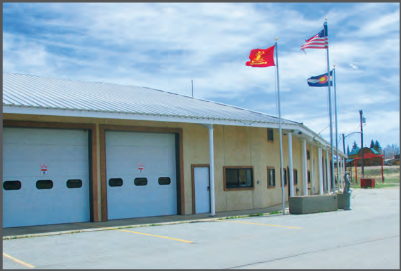
Wet Mountain Fire District Building in Westcliffe.
