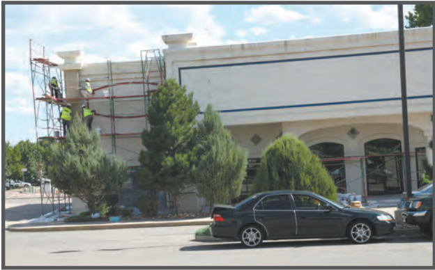
The work commences at Shops at Four-Mile Creek.
