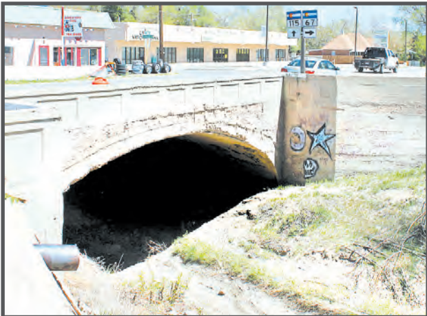
Historic Bridge on corner of Hwy 67 and Hwy 115 in Florence, Colorado. Photo from WikiMediaCommons,2013
